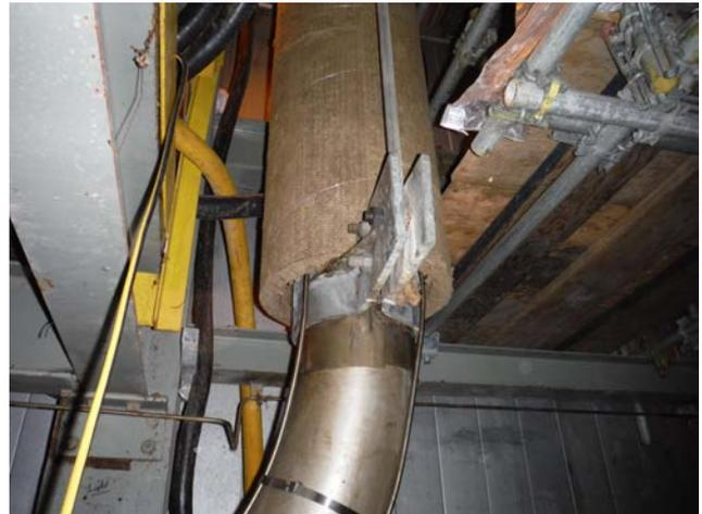
Also atmospheric corrosion phenomena from the outside of high-pressure piping can endanger the integrity of high-pressure pipeline systems in urea plants. During asset lifetime studies in urea and ammonia plants several times severe external corrosion was encountered.
