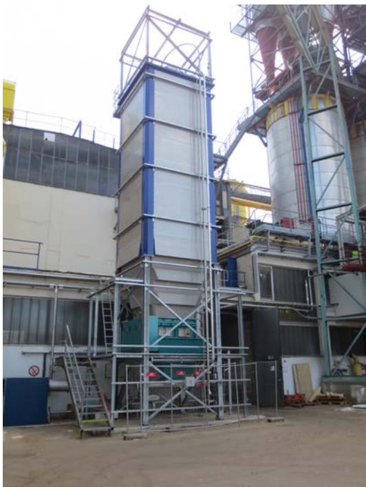
GEROLDINGER set itself this challenge and for the storage of 60 tonnes of urea (about 2 silo trucks) it created a space-saving, environmentally-friendly solution with an octagonal Multigon silo (65 m<sup>3</sup>). This special silo facilitates easier crust breakup thanks to its flexible walls and with the aid of the tried and tested “Oszillomat” system it permits an even discharge of the urea.
