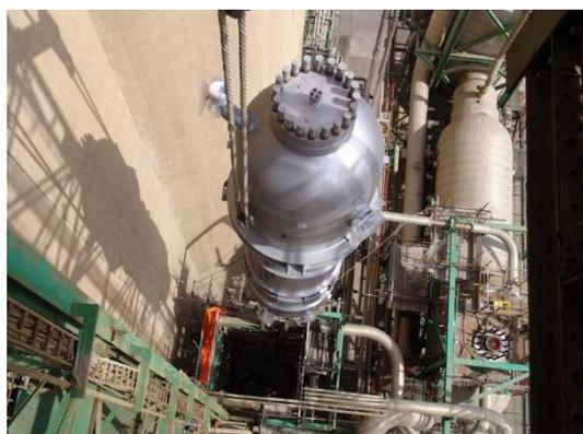
*Fig. 9: Equipment replacement during a revamp*
