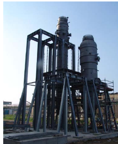
Picture 2: Replacement project at SKW
